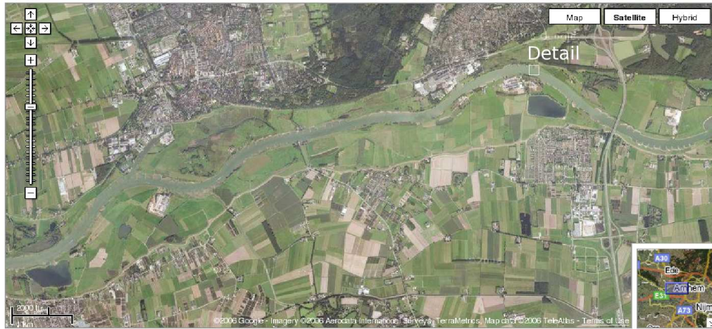
Figure 5.9: Satellite picture of the river part that is modelled in the Randwijk model and its surroundings.
