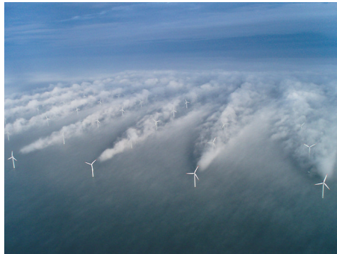
Figure 1.1: Wakes effects for Horns Rev 1 offshore wind farm at Denmark. Source: Christian Steiness
